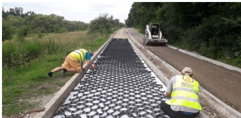
Fig. 2. Construction of the first part of the Green Line project in Ivan Pavel II Park. June 2022
